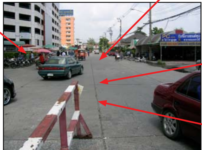
A straight-line road to the end of the site with no traffic-calming devices
